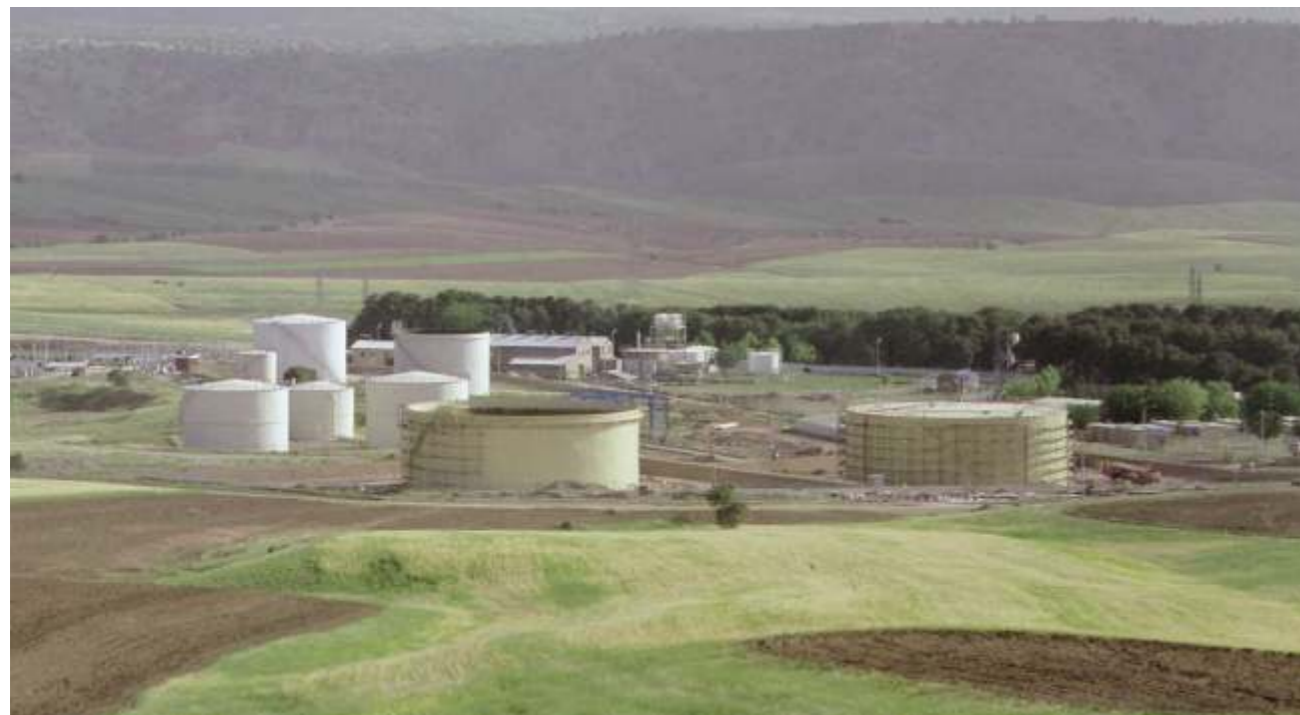
Khorram Abad Pump Station
